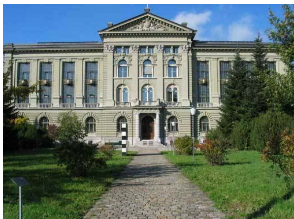
The building of the Swiss Federal Archives in Bern.
